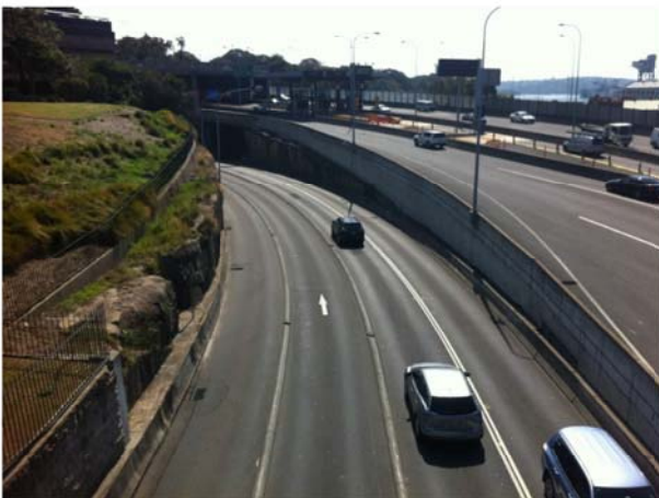
Photo 5: Looking north from the Wilson Street footbridge towards Sir John Young Crescent and the Eastern Distributor
